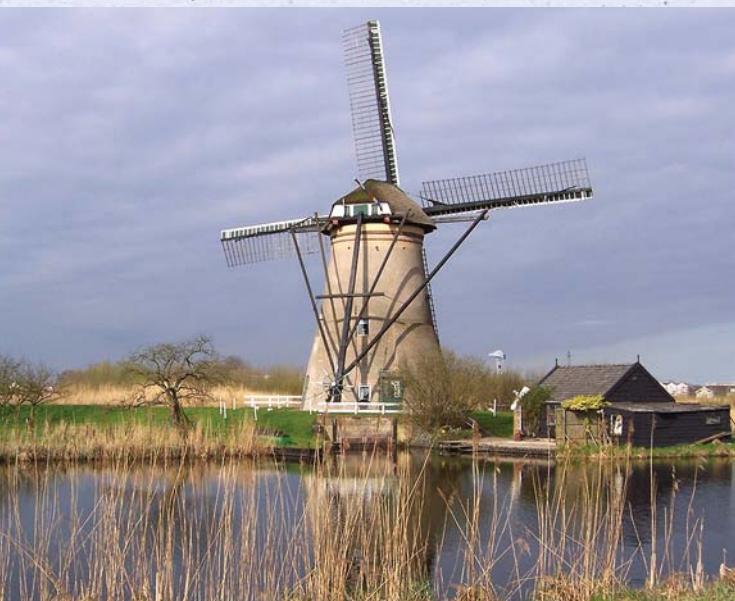
2nd Windmill at Kinderdijk, the Netherlands Pat Woods—Sun City West, Arizona
